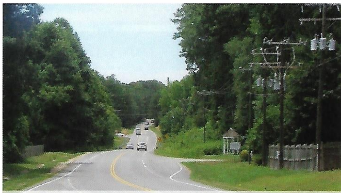
Existing Conditions—Looking West at Gladstone Glen Place
