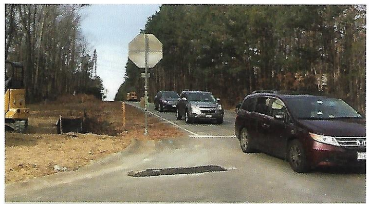
Existing Conditions—Looking West at Water Willow/Walton Bluff Pkwy
